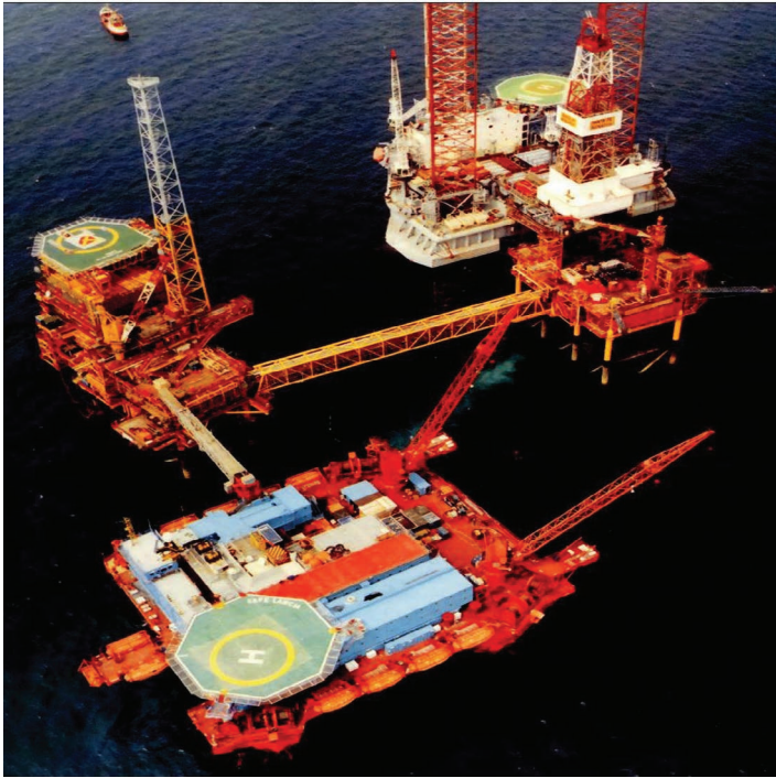
FIGURE 13.4 Ariel view of an offshore complex installation. Each platform is linked by covered companionways and has its own heli-pad landing facility. The drill tower is seen in the top right hand corner. All sections have local crange to receive relevant stores from offshore supply craft.
