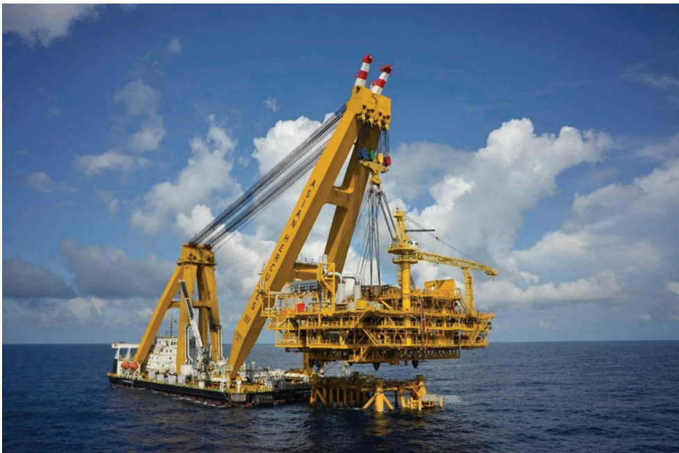
FIGURE 13.6 Asian Hercules II (IMO No. 8639297) a crane barge, floating sheerleg platform of the Asian Lift Pte Ltd, engages in a modular build up, to an offshore steel jacket of a developing offshore installation.
