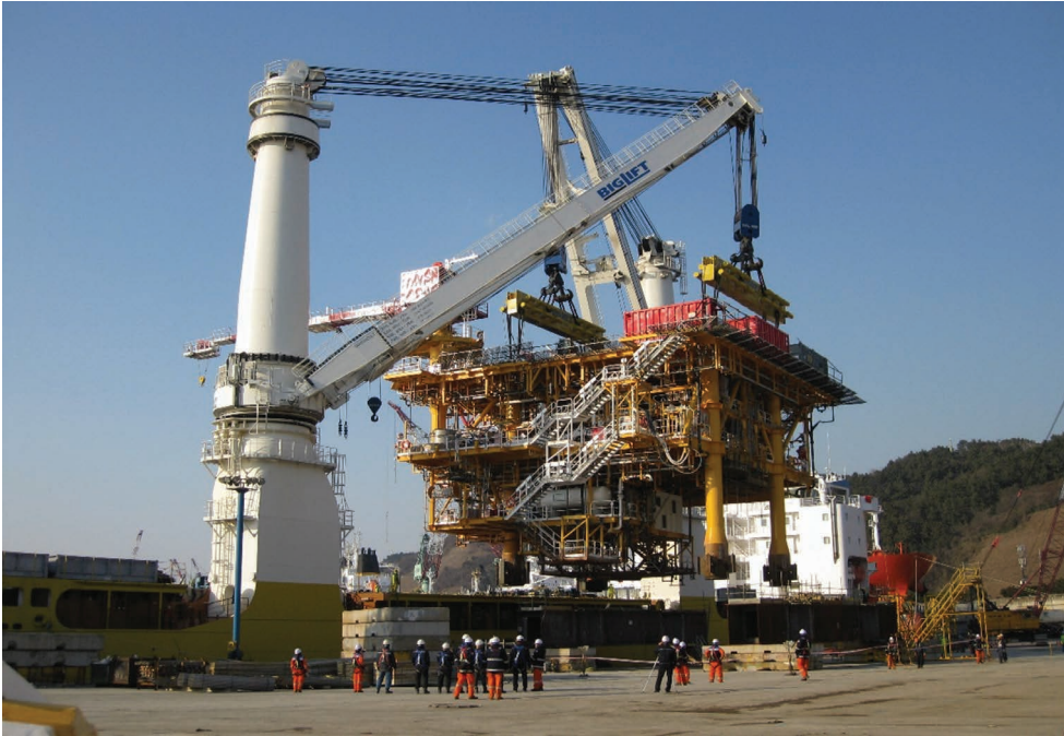
FIGURE 4.24 The 'Happy Star' (IMO No. 9661259) one of the Big Lift shipping company's vessels engages in lifting a topside module by means of heavy duty lifting beams and a tandem lift by its two on board Huisman heavy lift cranes.
