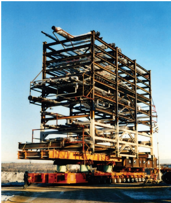
FIGURE 4.28 A Scheuerle multi-wheel transport platform, seen engaged in ground handling of a steel installation structure. The movement of such a load must be logistically planned, prior to the building/construction phase of the project.
