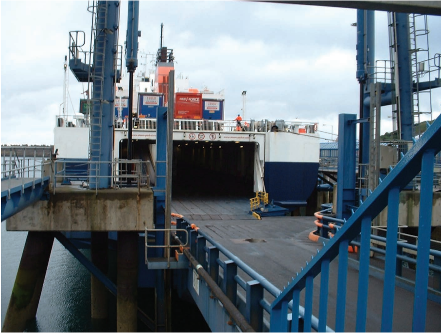
FIGURE 8.31 A typical road companionway adjustable link to a concrete structured dolphin at the port of Heysham, Cumbria. The height of the dolphin platform is built to accommodate the range of tide to allow acceptance of the vessels stern ramp. The ships stern door/ramp is then lowered for the angled flaps to lay flush to the companionway.
