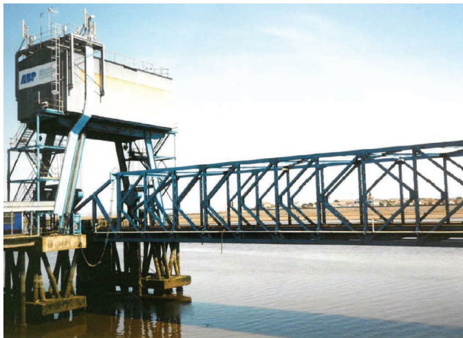
FIGURE 8.32 A typical mechanical link span machinery housing for hoisting and lowering the link span down to a position above the waterline. The stern ramp of the Ro-Ro ferry then lowers her stern ramp onto the links driveway to permit discharge of vehicles. The rise and fall of tide of 10.5 metres is countered by the adjustment of height to the link span to allow continuous operations no matter what state of tide.
